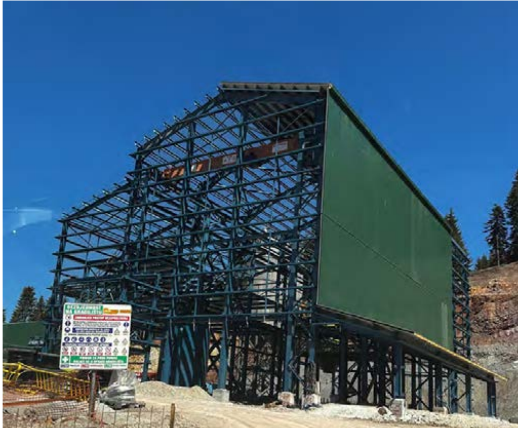
Construction of paste backfill plant advancing well
