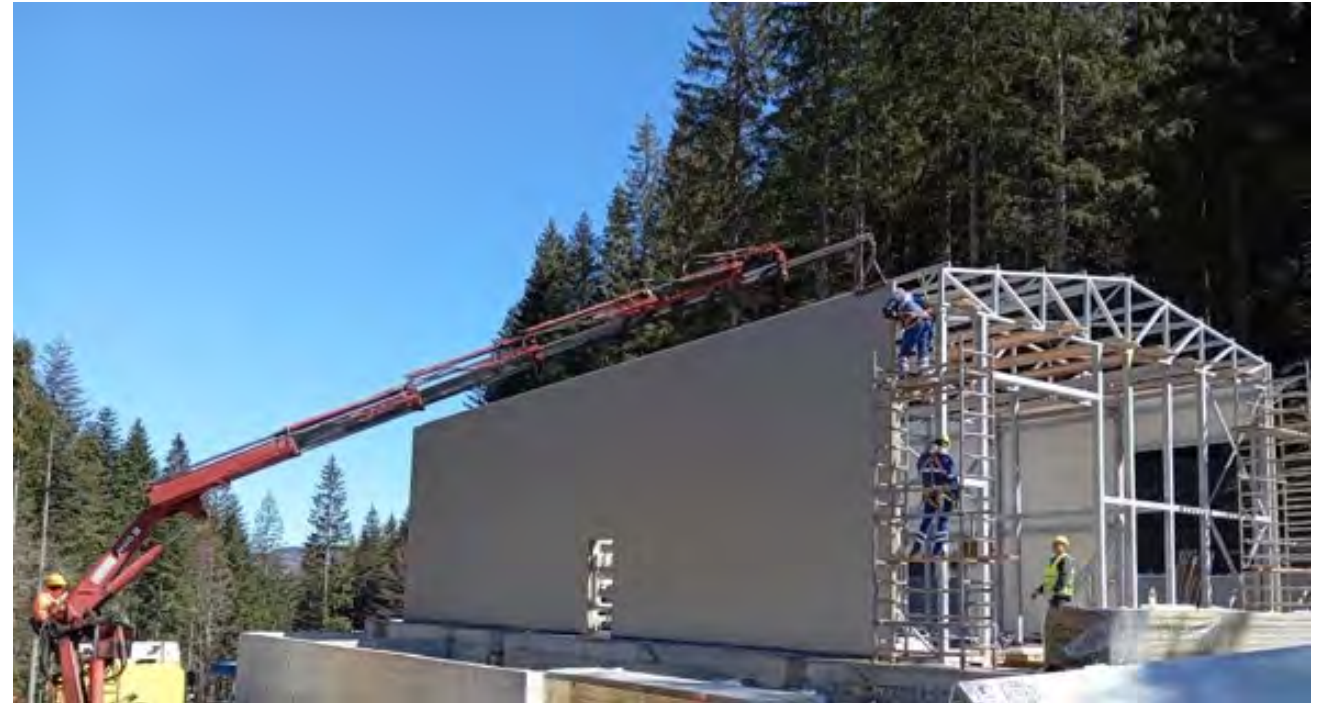
Installation of the water treatment plant
